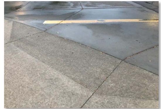
Corte Sierra non-ADA compliant ramps
