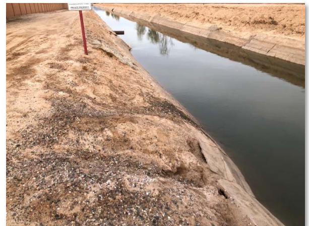
Canal lining eroding
