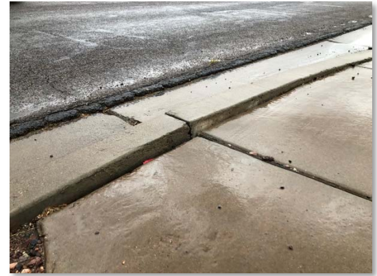
Corte Sierra sidewalk foundation issues
