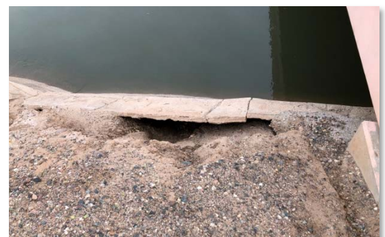
Canal lining eroding near the bridge south of Osborn Road and Santa Fe Trail
